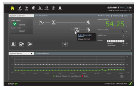
STATUS OF DC/DC CONVERTERS IN SMARTPACK2 WEB
