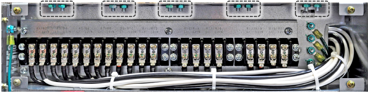
Figure 3 - AC Ground Connections
