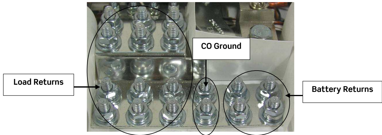
Figure 8 - Recommended Return Bus Organization
