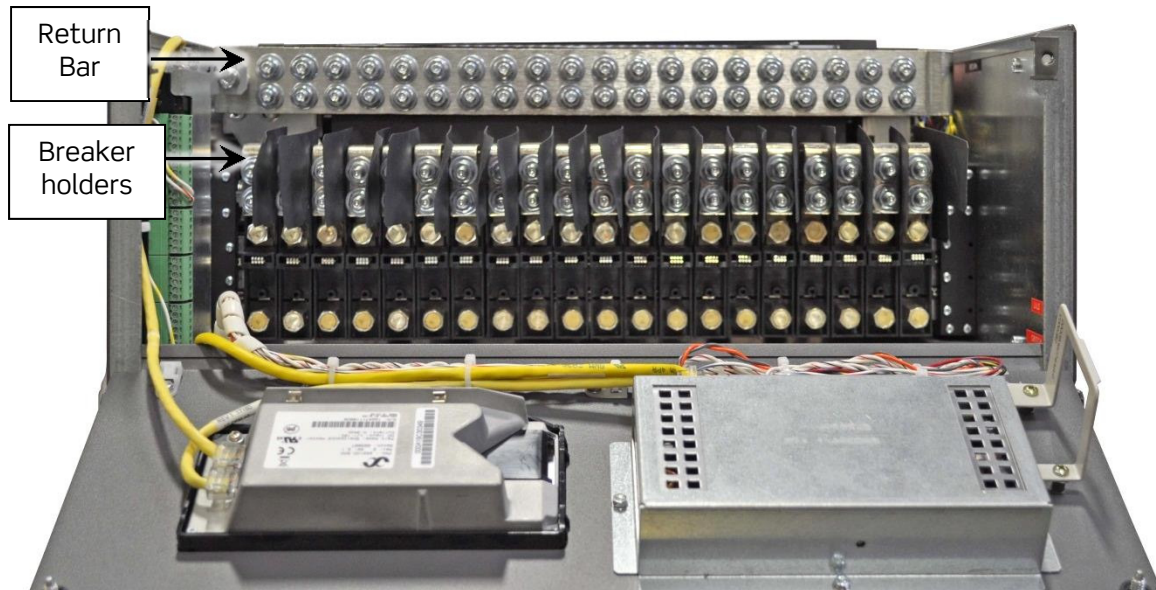
Figure 24 - Distribution with Adjustable Breaker Holders
